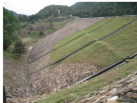
Saraphgarh Earth Dam
