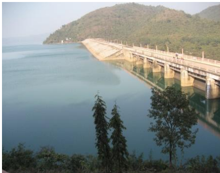
Salandi Hadgarh Dam
