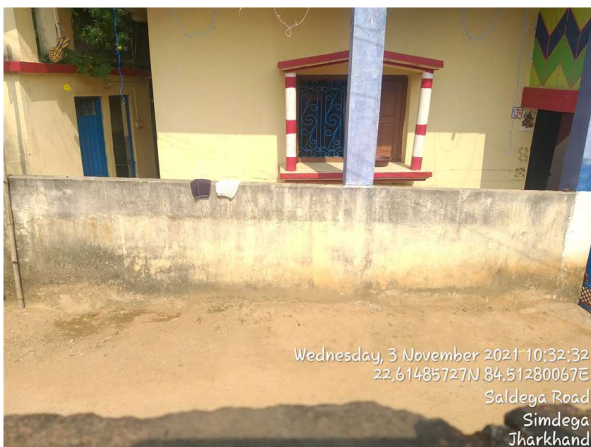
Wednesday, 3 November 2021 10:33:24 22.61485974N 84.51272952E Saldega Road Simdega Jharkhand
